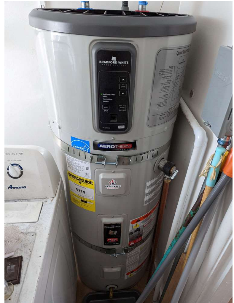
Heat pump hybrid water heater
